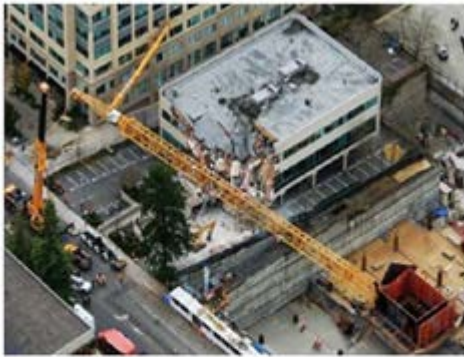
The scene the morning after a construction tower crane collapsed due to a foundation problem. One person was killed and several buildings were damaged.
