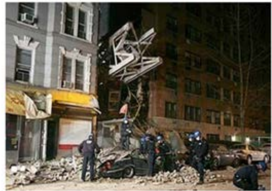
This 19-story crane broke away from an apartment tower while being prepared for jumping. During the lifting of the climbing assembly/section, the rigging failed, causing the section to fall and damage the building ties and the crane to fall. Six construction workers, including the crane operator were killed, along with a tourist visiting the city.
