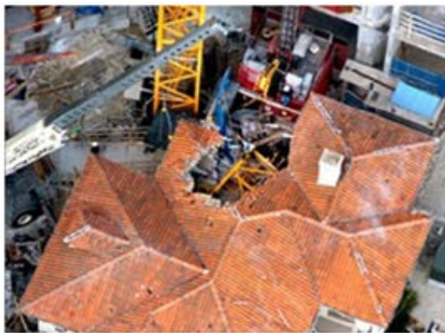
During preparations for jumping a construction tower crane, a 20 foot long tower section of the crane plummeted 30 floors at the site of a high-rise condominium, killing two workers and smashing into a home that the contractor used for storage. Five other workers were injured.
