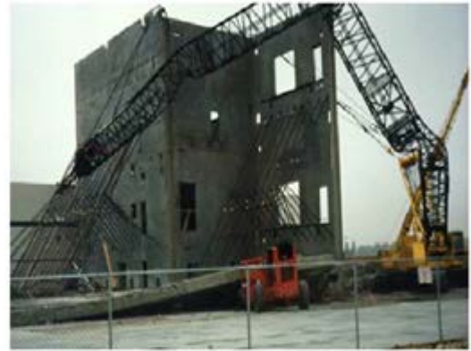
Another accident that occurred while lifting pre-cast concrete panels. The load contacted the boom, causing the boom to fall.
